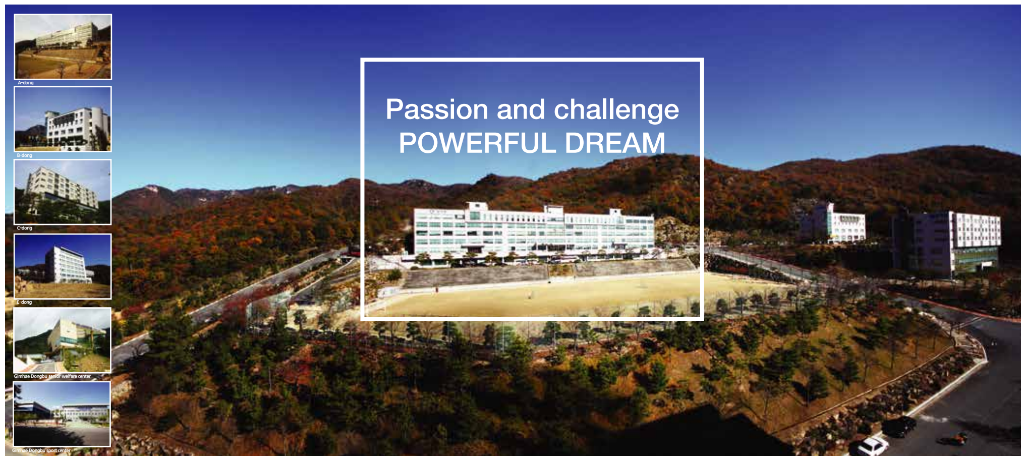
View of campus view from E-dong
